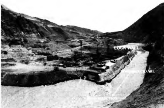
Fig. 10: Photograph showing full phase diversion
