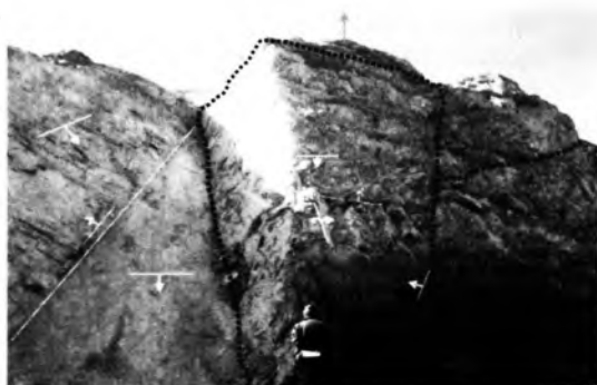
Fig. 9: Photograph showing slip plane after failure
